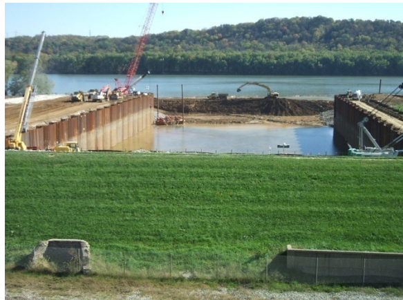
Ground level view of OPEN CELL structure
