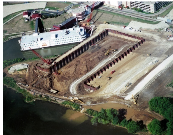
Over 4,100 tons of flat web sheet pile were used during construction
